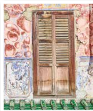
Façade of 66 Spottiswoode Park Road, oldest painted façade in Singapore
